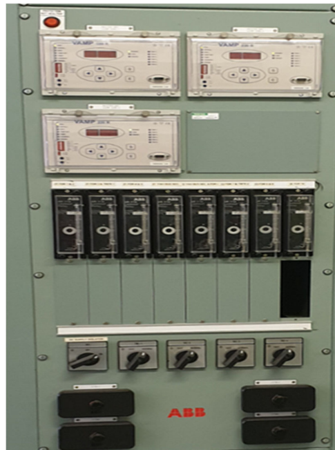
Figure 2: Existing Vamp Protection Panel
