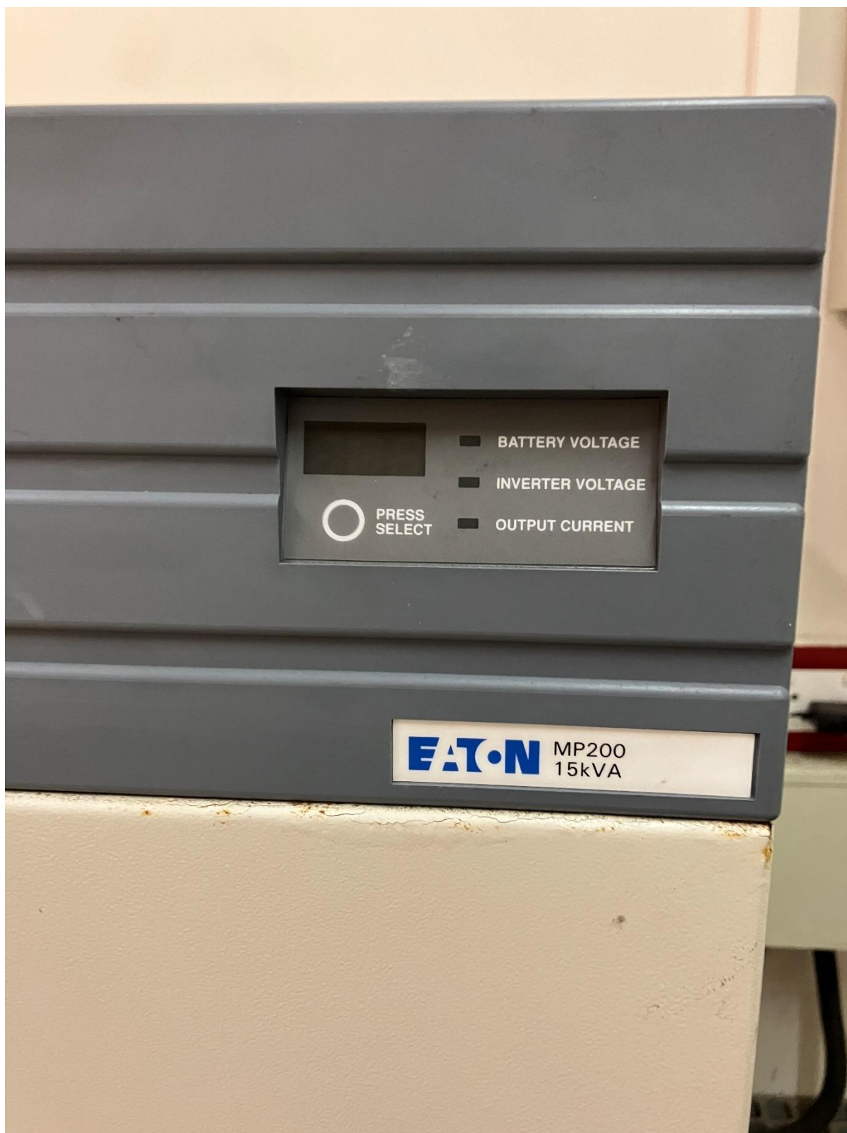
Faulty Eaton 15 kVA UPS in LV Room
