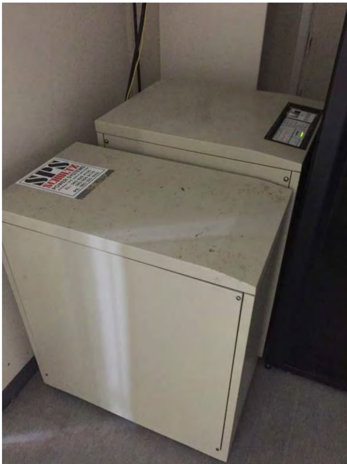
Conference Centre Existing UPS Image 1
